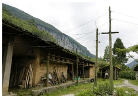
No Electricity Areas
